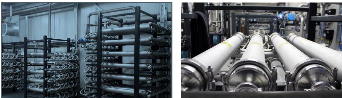
Rys. 3k. System membran do uzdatniania biometanu
